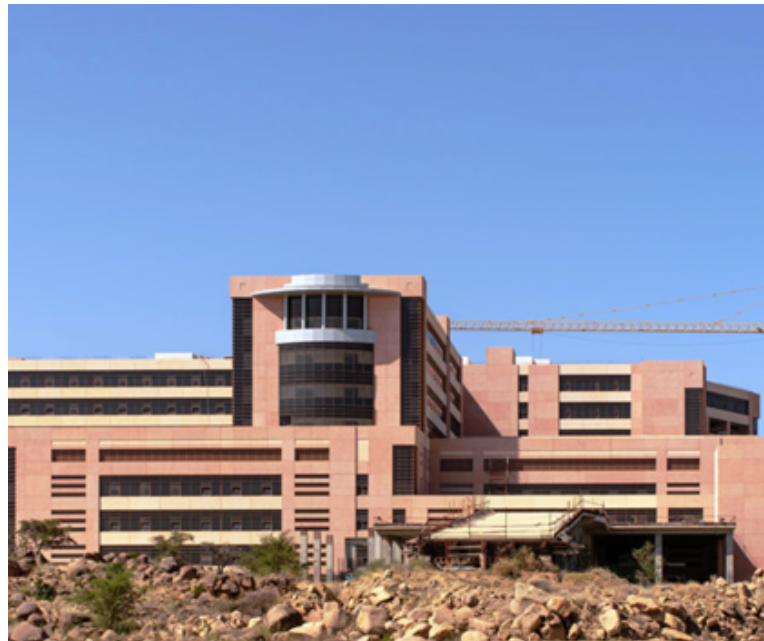
KING KHALID UNIVERSITY HOSPITAL (KKUH)
